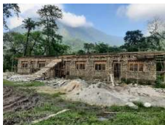
BHU staff quarter at Piping
