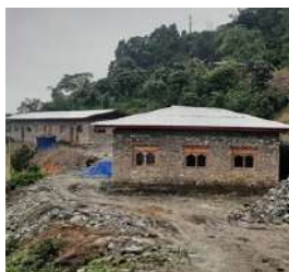
Construction of BHU II at Kamji
