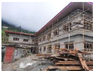
Staff quarter construction at Gedu
